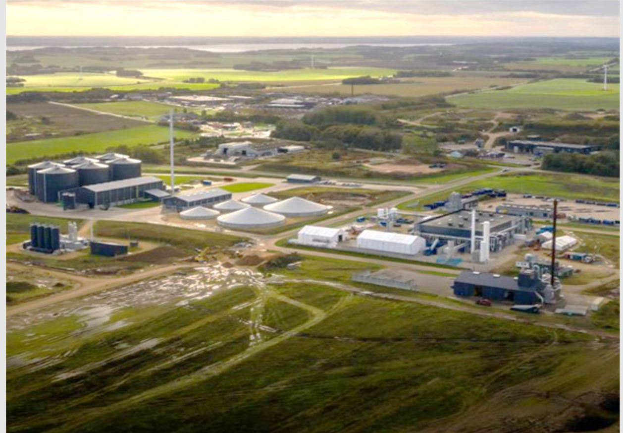
Illustration: Biogas and coming PtX plant: GreenLab Skive
