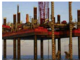
e) Towed jack-up crane barge
